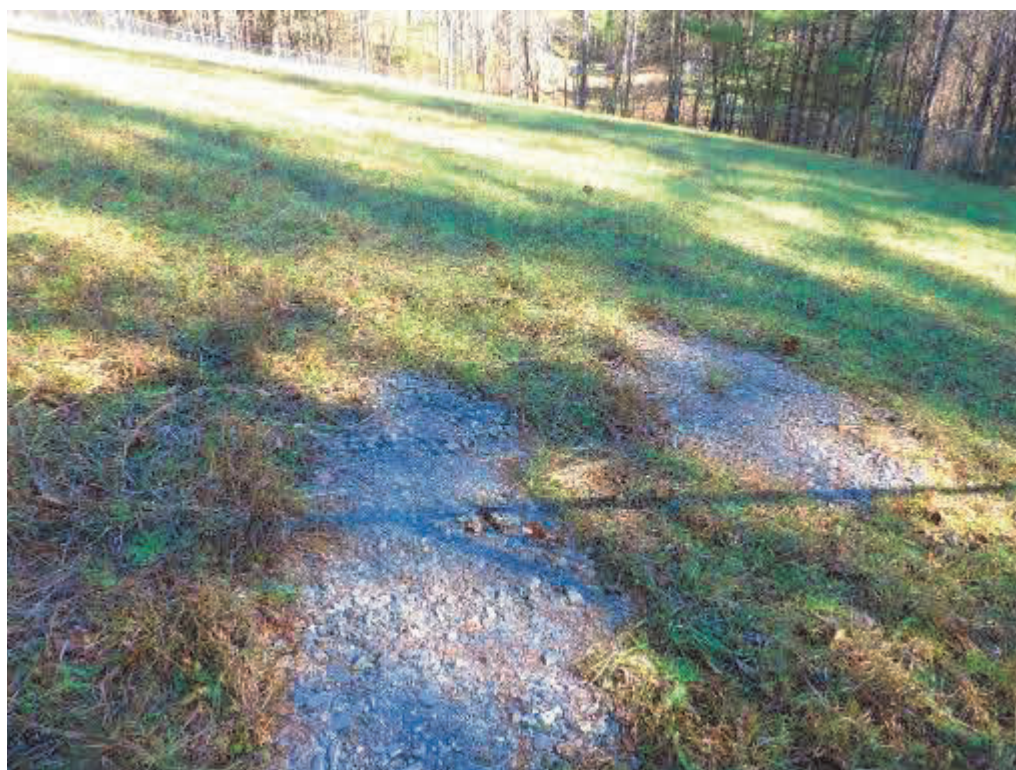
Areas filled with gravel to address bears digging on the surface of DA-7/8 (BV)
