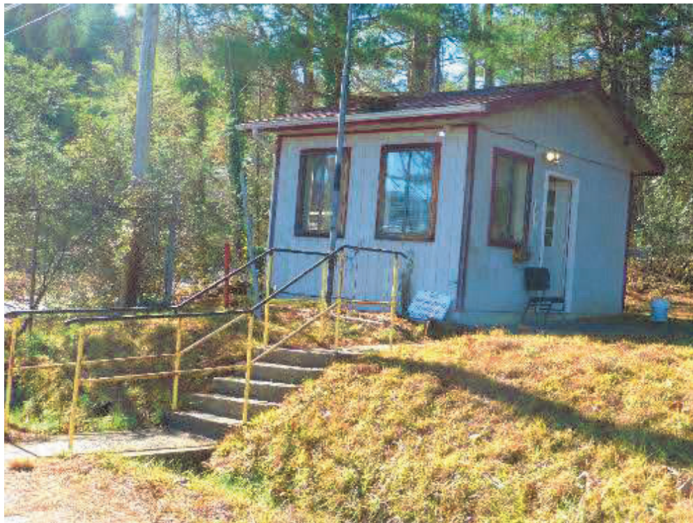
Security guard hut at front entrance gate
