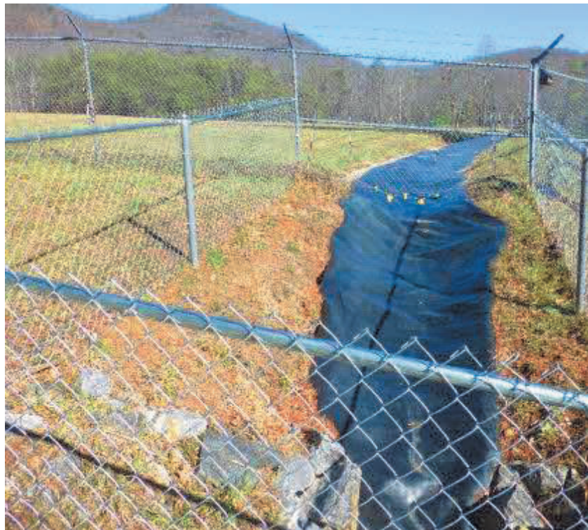
APA stormwater diversion swale discharge area
