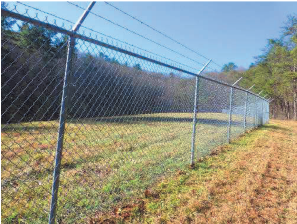
Fence and cap at DA-10/11 (FV)
