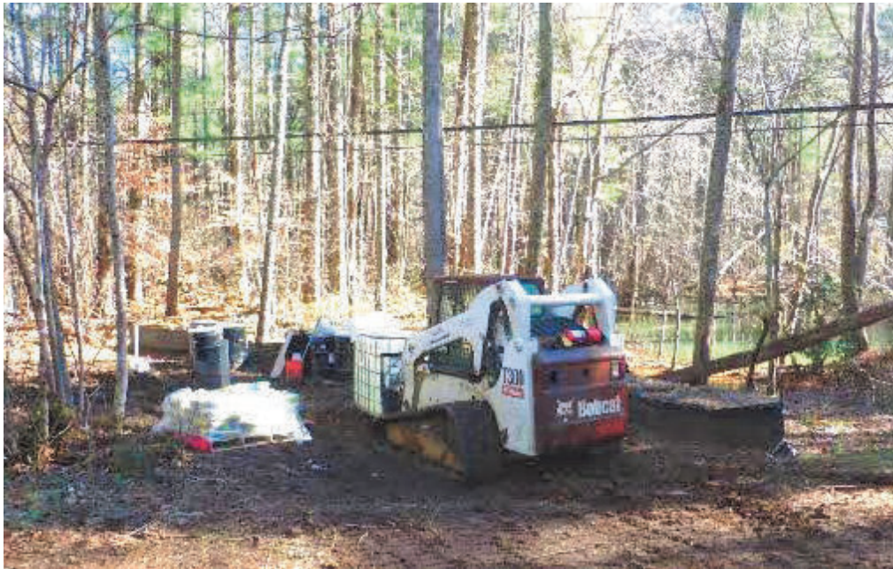
Installation of new BV wells downgradient from the MW172-T32D area (this downgradient area of new well installation is referred to as “the Narrows”)
