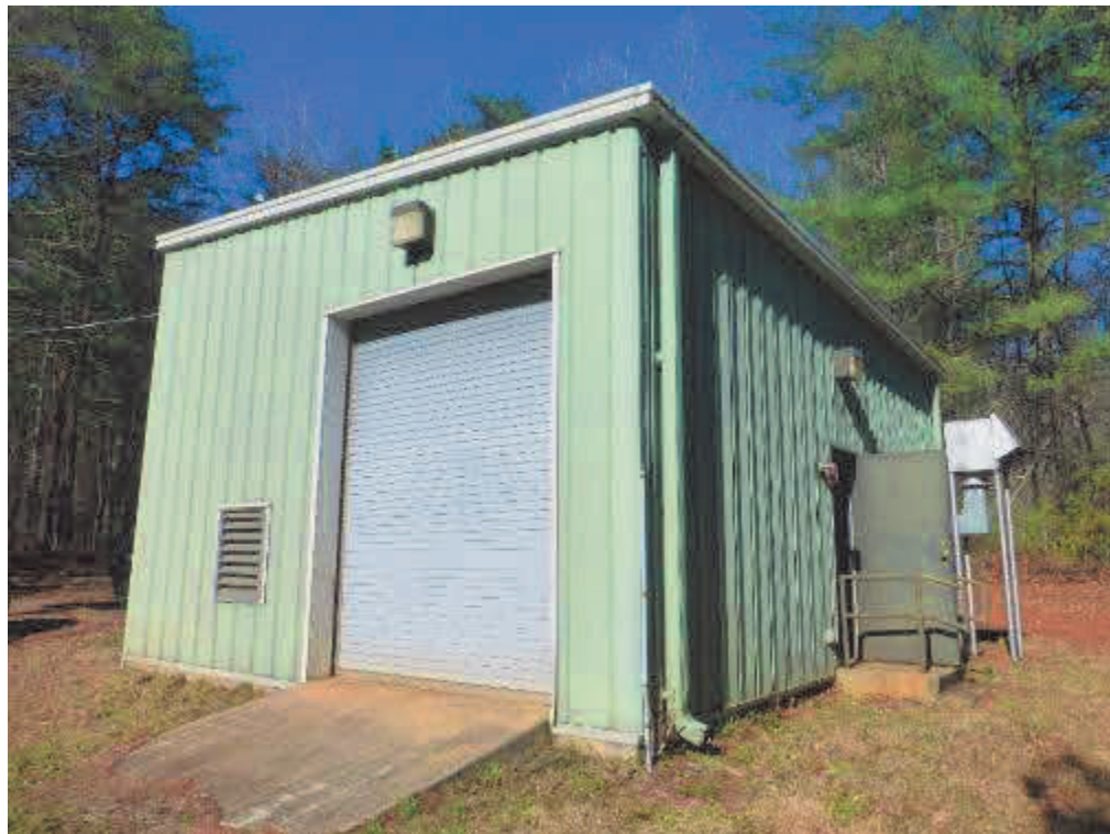
Exterior of the BV groundwater treatment system building
