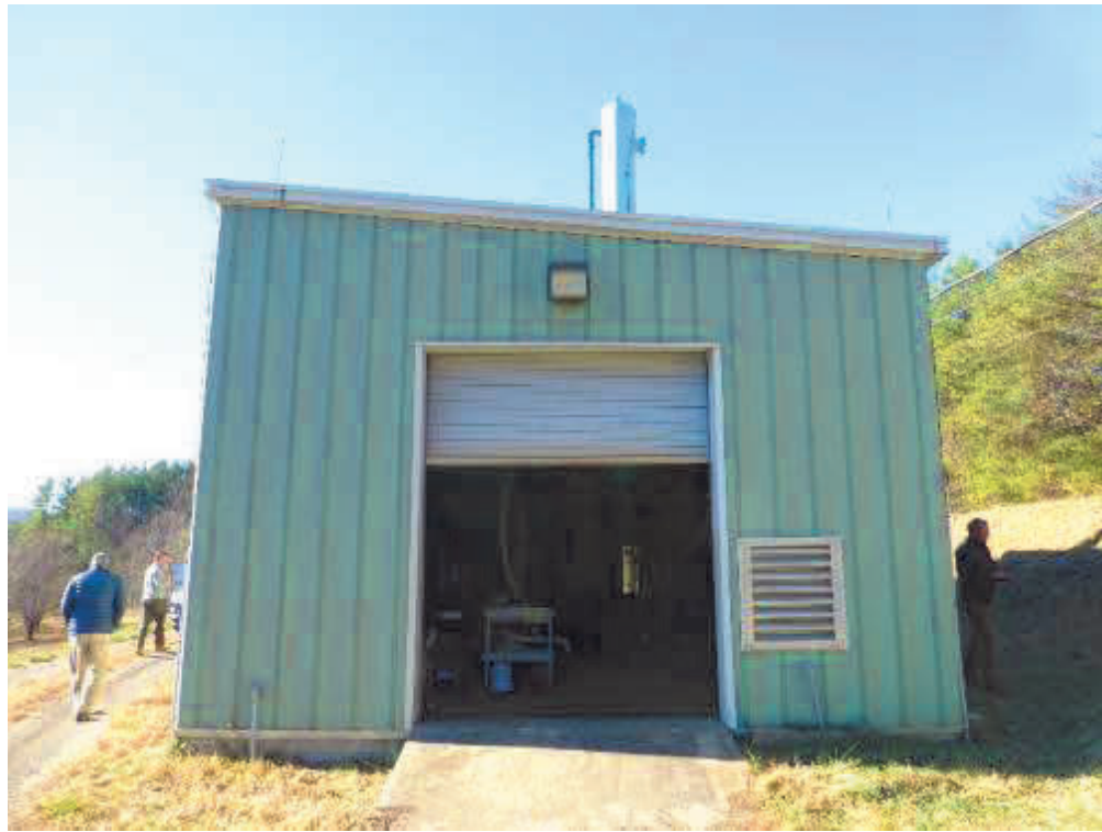
Exterior of the FV groundwater treatment system building
