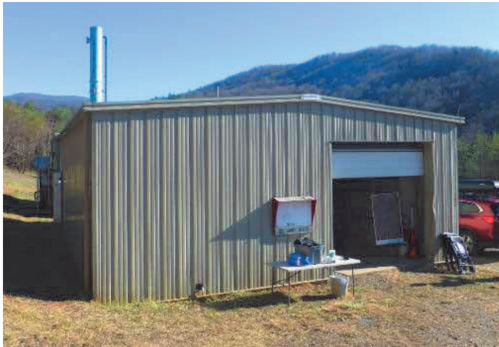
Exterior of the FV maintenance shed
